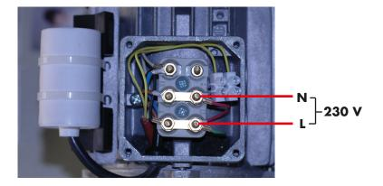
Motors controlled by MicroStart are single-phase motors wired for 1x230 V. An operating capacitor is used to assist start. The capacitor is located either in the MicroStart control unit or the motor. Also refer to the MicroStart connection instructions.
